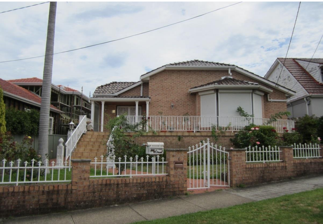
Figure 21: 6 Rodd Road, Five Dock – current
