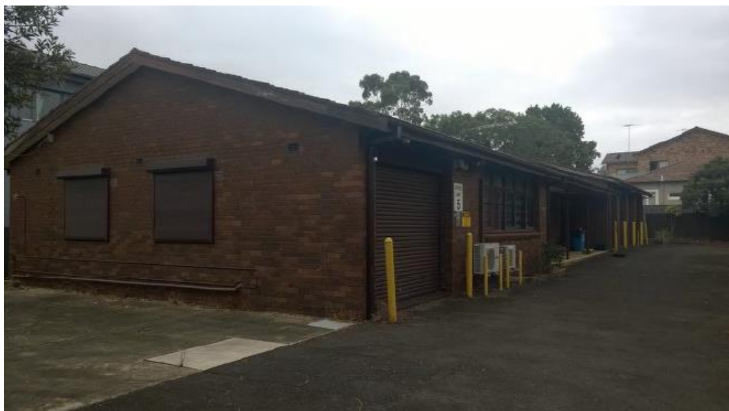
Figure 29: Depot Building (Lot 95 DP 6743) – building has recently been demolished
