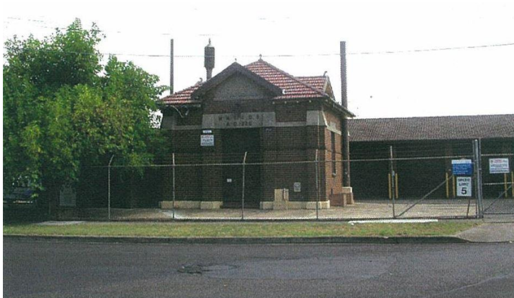
Figure 28: MWS & DB Pumping Station – 32 Wymston Parade 2007
