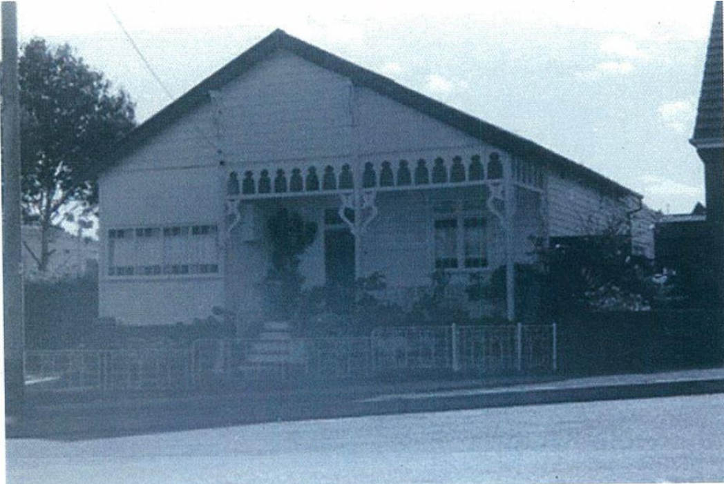
Figure 20: 6 Rodd Road, Five Dock – 1996
